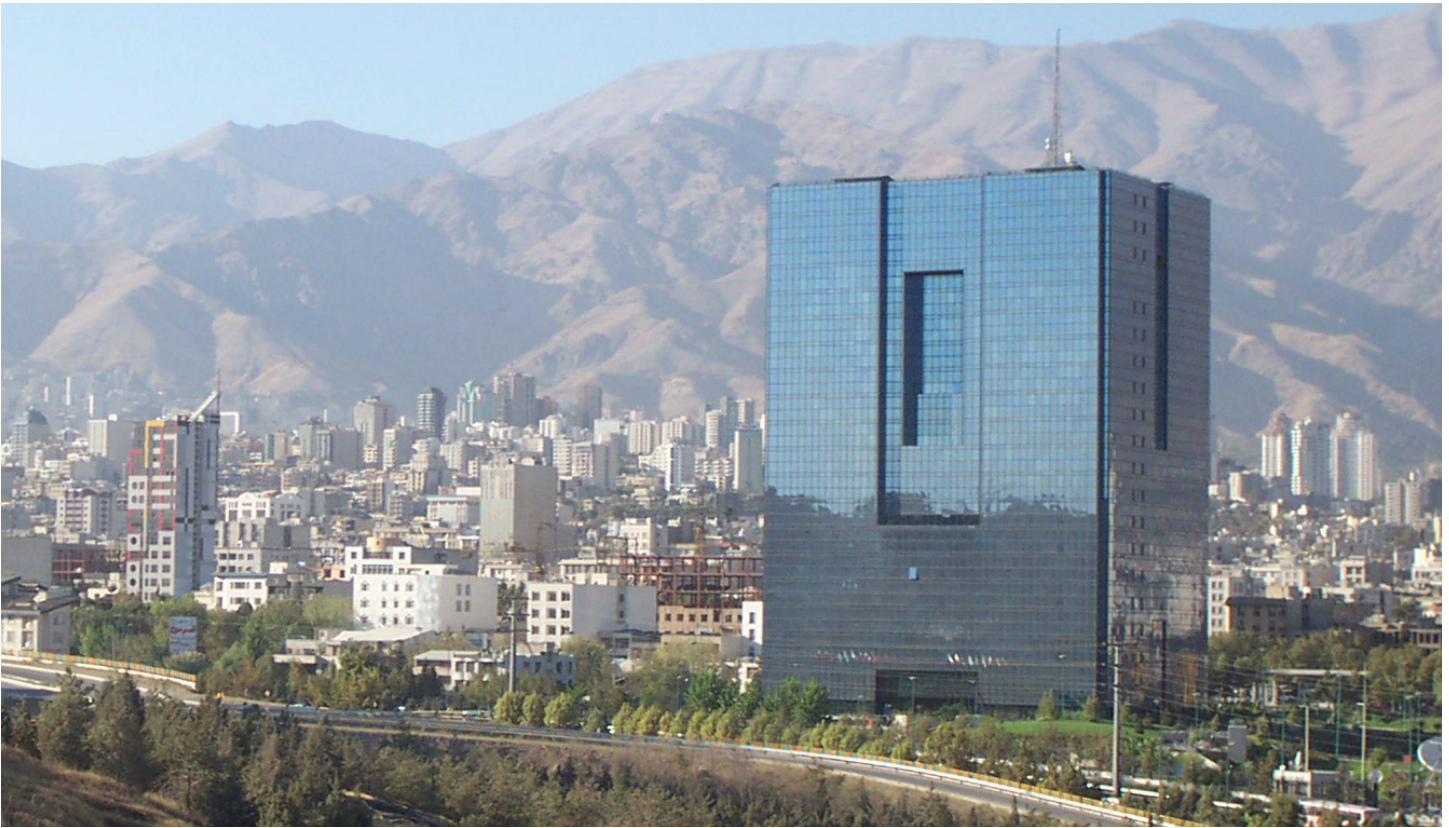
Bank Markazi (the Central Bank of Iran) on Mirdamad Boulevard, Tehran, Iran. Photo credit: Flickr/Ensie & Matthias.
