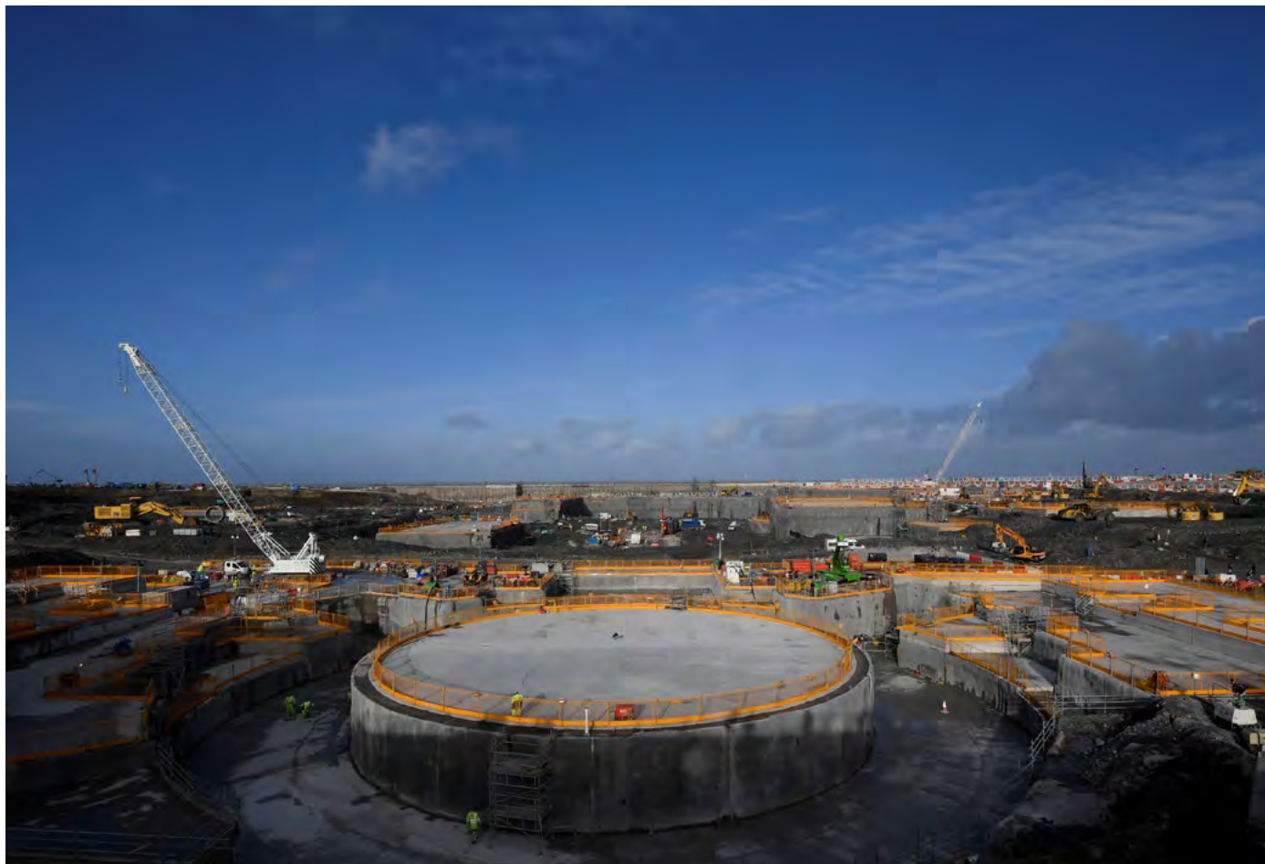
Construction including one of two 'nuclear islands' is seen at the Hinkley Point C nuclear power station near Cannington in southwest England, January 17, 2018. Source: REUTERS/Toby Melville.
