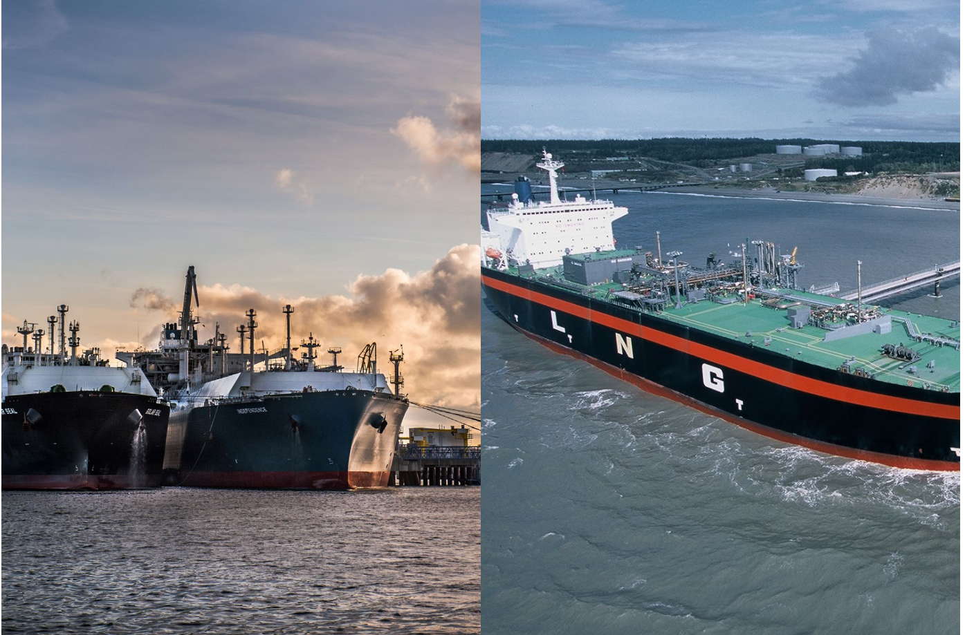
Substitution of non-Russian sources will enhance European energy security. Left: The liquefied natural gas (LNG) terminal in Klaipeda, Lithuania. Photo credit: ©KN. Right: LNG Tanker in Kenai, Alaska. Photo credit: ConocoPhillips Company.
